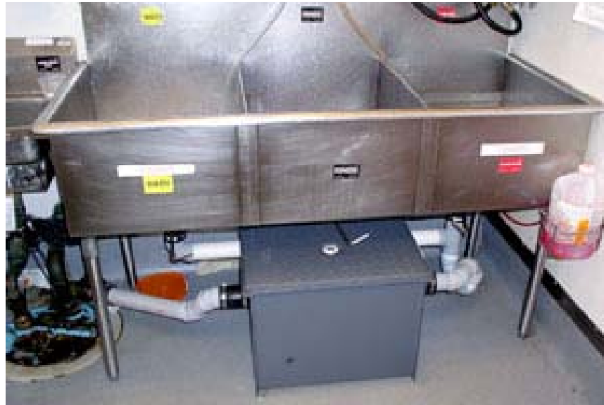
A 20 GPM, 40 lb hydro mechanical grease interceptor
